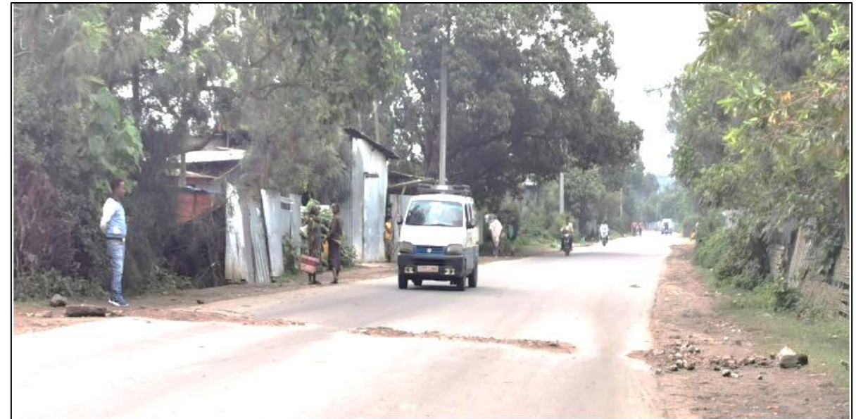
Figure: Speed bumps made by local people on Wendogenet Road, Ethiopia (Source: WRI, Ethiopia)
