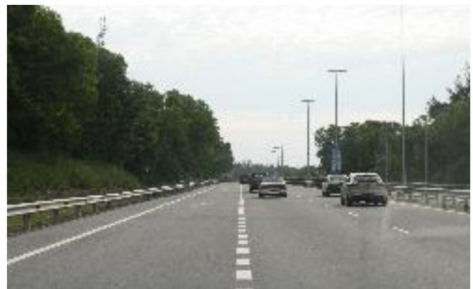
Figure 6.79: Well defined acceleration lane—Brunei.
