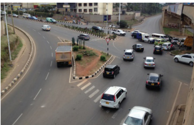
Figure 6.67: Wide-angled slip lane with poorly aligned crossings and lack of crossing.
