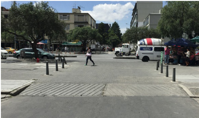
Figure 6.48: Raised intersection in Bogotá to give priority to pedestrians on an arterial street.
