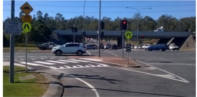
Figure 6.69: Raised crosswalk on slip lane with ghost island markings and crosswalk signs.
