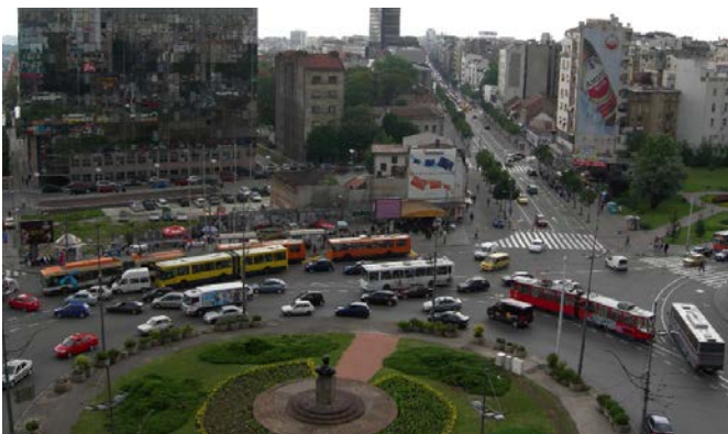
Figure 6.39: Roundabout (rotary) with improper lane alignment and width creating extra lanes in Serbia.
