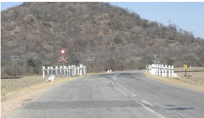
Figure 6.87: Rural rail crossing—Zimbabwe (passive).
