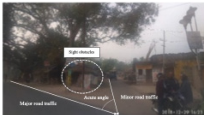
Figure 6.1: Uncontrolled Y-intersection in India.
