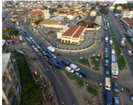
Figure 6.62: Poor delineated slip lane in Ghana.
