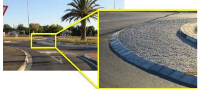
Figure 6.37: Truck apron with correct design for use by trucks only with a narrow circular carriage in South Africa.
