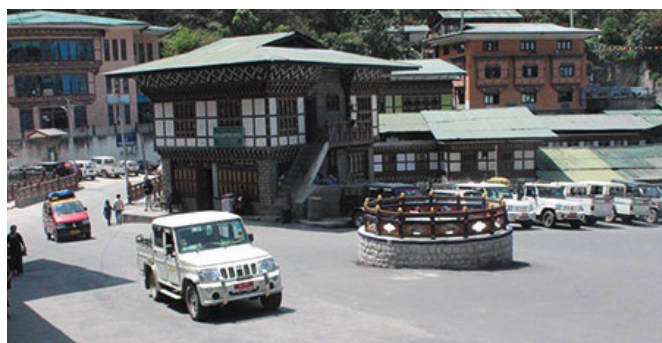
Figure 6.35: Inappropriate location and size of roundabout in Bhutan.
