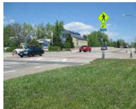
Figure 6.53: Raised intersection with crossing sign.
