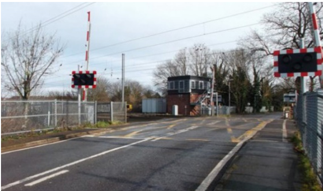
Figure 6.85: Rail crossing UK.
