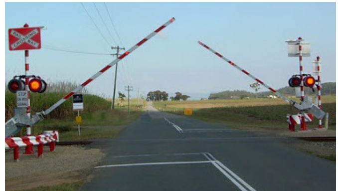
Figure 6.88: Rural rail crossing—Australia (active).
