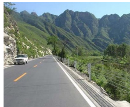
Figure 5.37: Cable barrier on tangent section.
