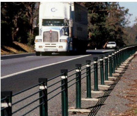
Figure 5.80: Flexible (wire-rope) barrier.
