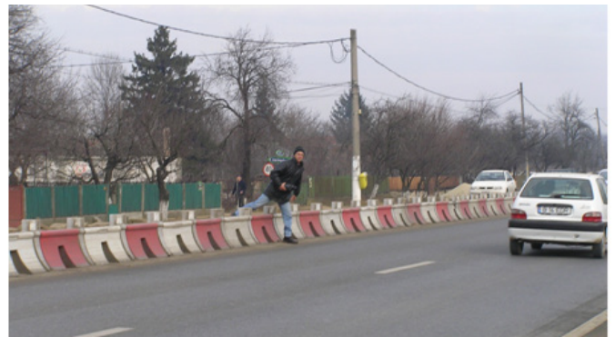
Figure 3.26 Poorly designed median for no crossing location—Romania.
