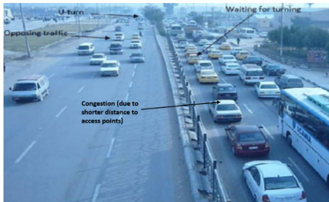
Figure 5.108: U-Turn on narrow median (with waiting lane).
