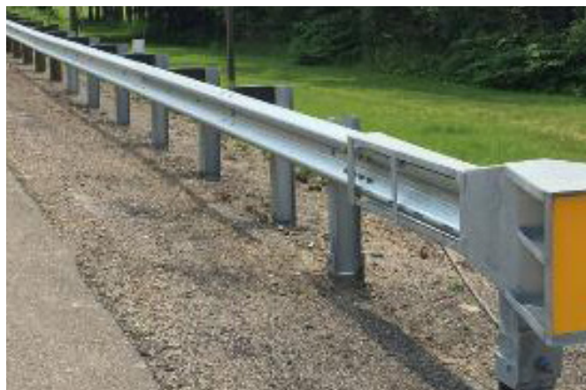
Figure 4.53: Typical metal barrier.
