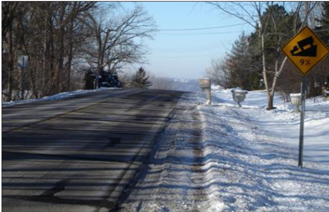
Figure 5.48: A steep grade warning sign along a road that appears to drop off in the distance.
