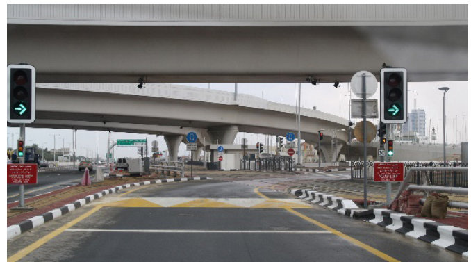
Figure 6.86: Automatic signal controlled crossing—Dubai tram.
