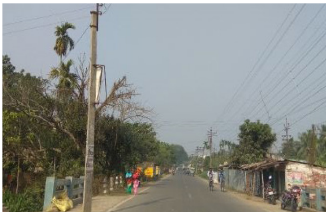
Figure 5.70: Rigid mast on shoulder.
