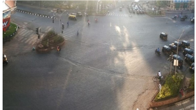
Figure 2.26: Before the HP intersection improvement in March 2017.
