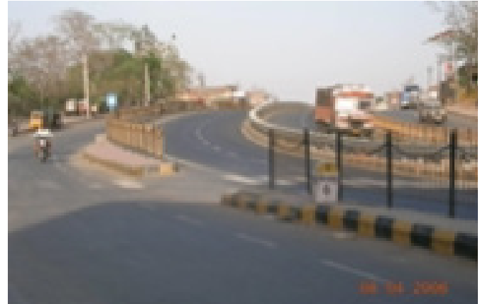
Figure 5.113: Use of nonstandard median type and unsafe median opening on a high-speed road.
