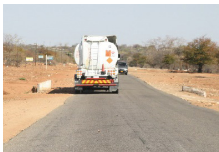
Figure 5.130: Typical culvert headwall to be extended/replaced.
