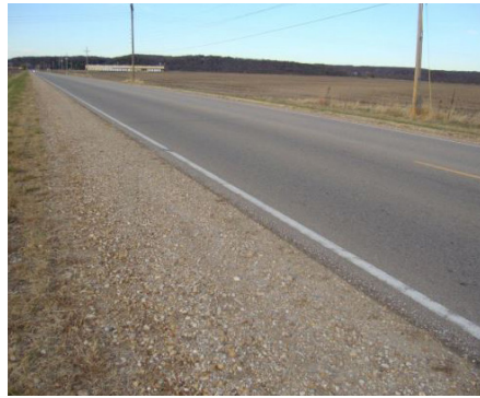
Figure 5.7: Unpaved gravel shoulder.
