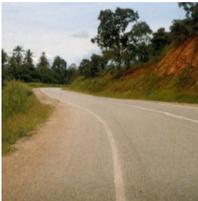
Figure 5.38: Example of introduced superelevation on curve
