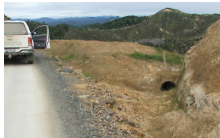
Figure 5.133: Piped flume.
