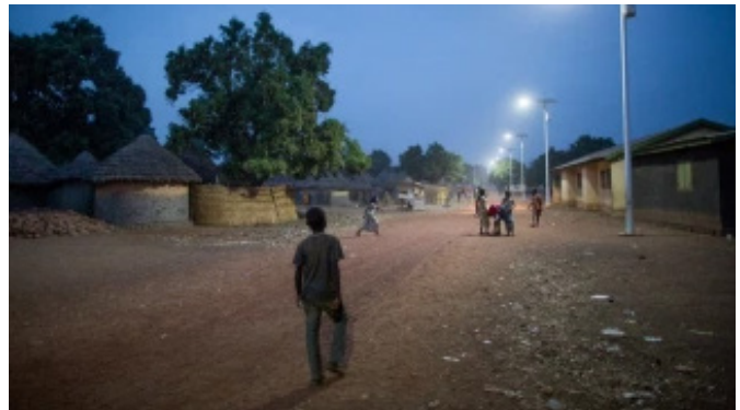
Figure 5.168: Solar powered streetlights.,
