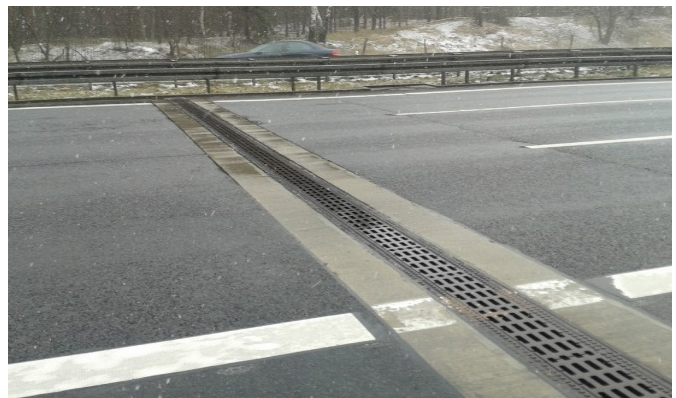
Figure 5.146: Transverse gutter.
