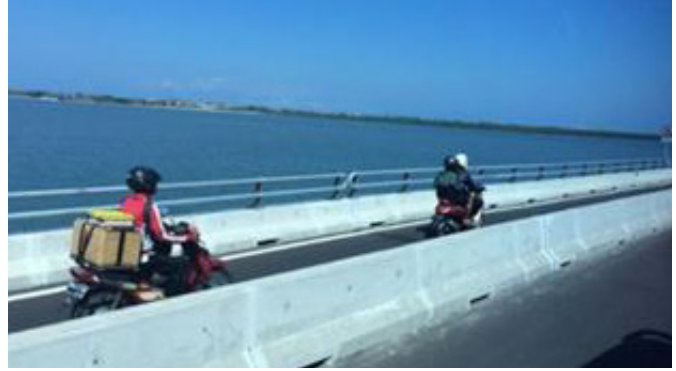
Figure 4.56 Modified U-shaped posts and attached to a curved concrete barrier
