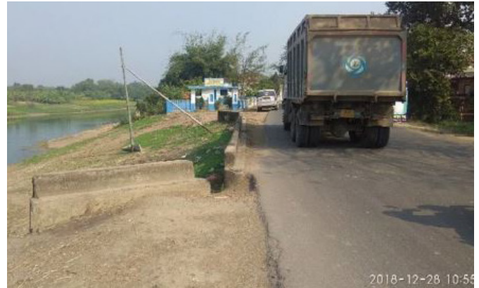
Figure 5.67: Unshielded water body with steep embankment.
