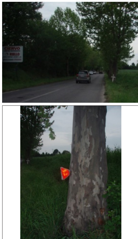
Figure 5.78: Roadside tree delineated but inconspicuous—Italy.
