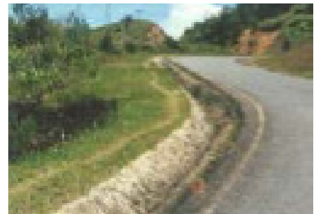
Figure 5.128: Conventional v-shaped drainage.
