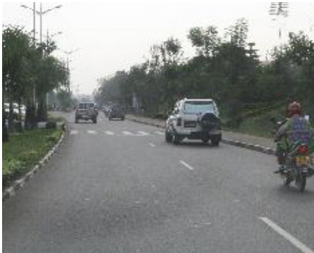
Figure 4.20: Well defined at-grade crossing—Rwanda.
