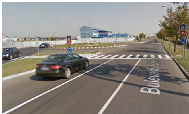
Figure 6.31: Dangerous roundabout design in Romania, where the main road has no deflection.
