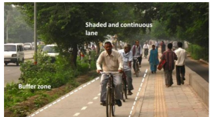
Figure 3.41: Walking and cycling facilities with buffer zone.
