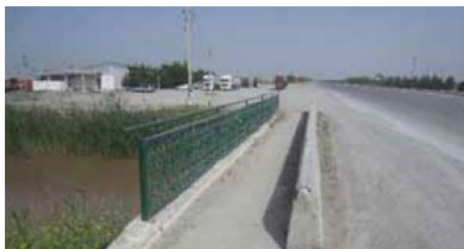
Figure 5.86: Light-gauge rails with concrete curbs.
