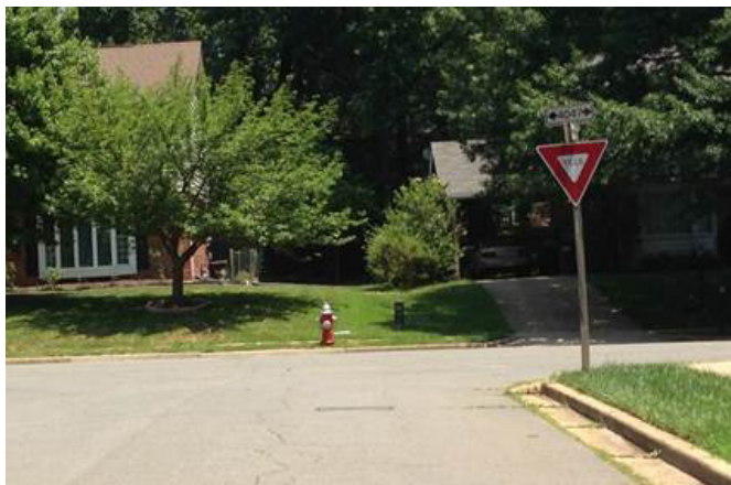
Figure 6.3: Yield signs being used as intersection control.
