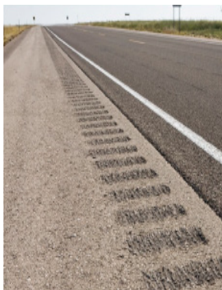
Figure 5.31: Shoulder rumble strips.
