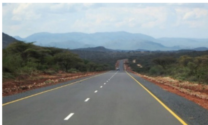
Figure 5.120: An asphalt road surface in good condition.
