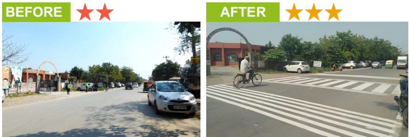
Figure 4.47: Installing crossings with advance cycle stopline—India.
