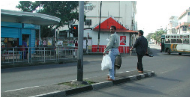
Figure 4.25: Lack of pedestrian space on median—mauritius—safety inspection.
