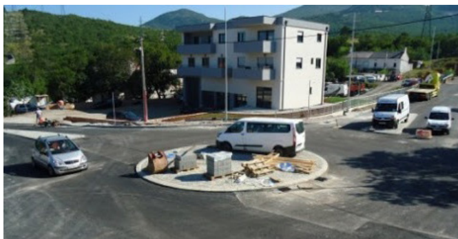
Figure 6.32: Vehicle ignoring flat roundabout in Croatia
