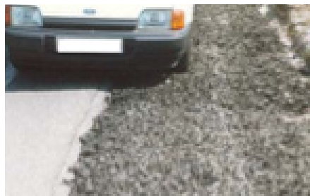
Figure 5.127: Closed drainage filled in with porous materials for anti-erosion and falling.,
