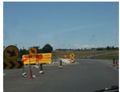
Figure 3.45: Well signed and controlled site—Tanzania
