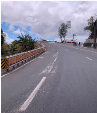
Figure 5.91: Fully re-directive crash cushion—Philippines.
