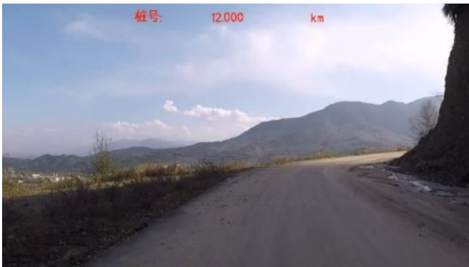
Figure 5.18: Insufficient delineation at curve.
