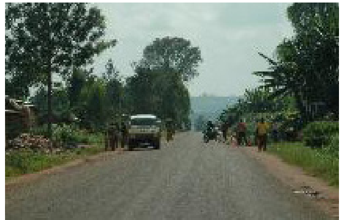
Figure 4.66: Rural village bus stop—Burundi, no signs or facilities.
