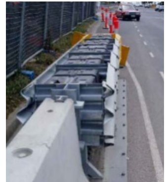
Figure 5.94: Safe crash cushion at the end of rigid barrier at a construction site.
