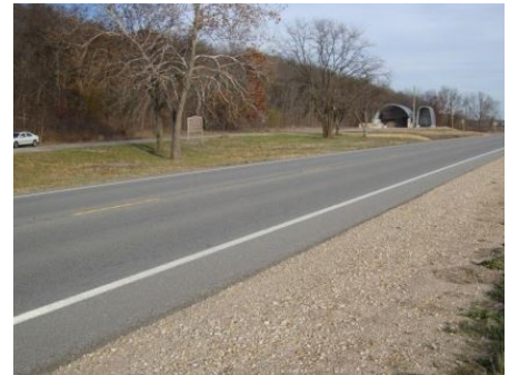
Figure 5.8: Partially-paved or composite shoulder
