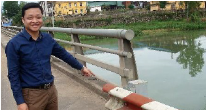
Figure 5.87: The exposed end of the guardrail can spear through an impacting vehicle.
