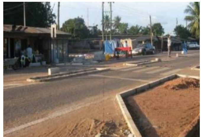
Figure 3.3: Road narrowing with traffic islands and extended curbs.
