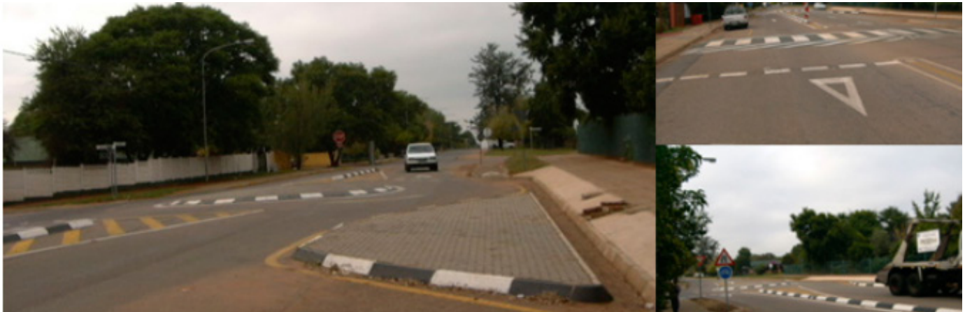
Figure 3.11: Use of mixed traffic calming infrastructure—narrowing, speed humps, and delineators
