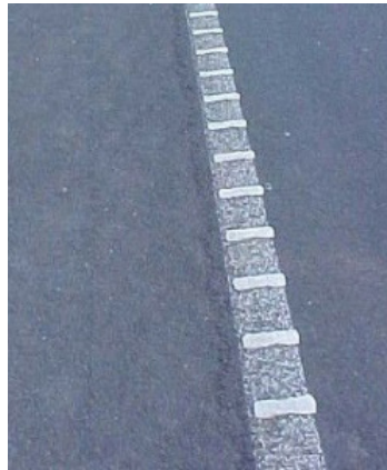
Figure 5.32: Edge line rumble stripes by adding ribs.
