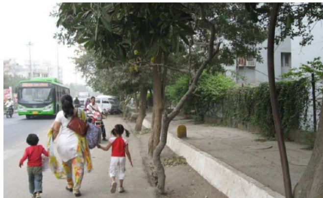
Figure 5.151: Very high curb (approx. 250 mm) limiting access by pedestrians to the walkway.
