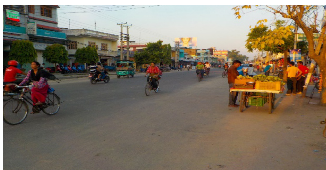
Figure 2.7: Stalls on the road with no separation of through high-speed traffic movements and mixed activity area—Nepal.
