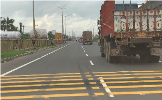
Figure 3.4: Rumble strips on highways.
