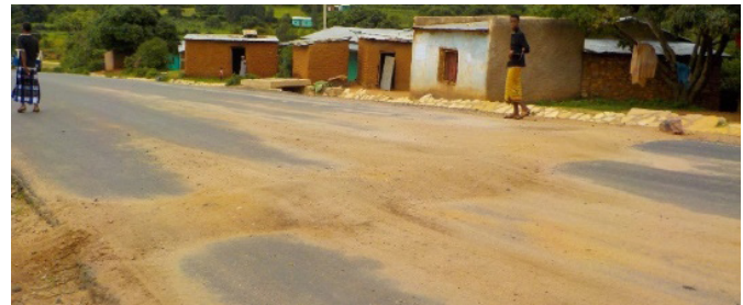
Figure 3.5: Speed bump placed by community on road passing through village—Ethiopia.
