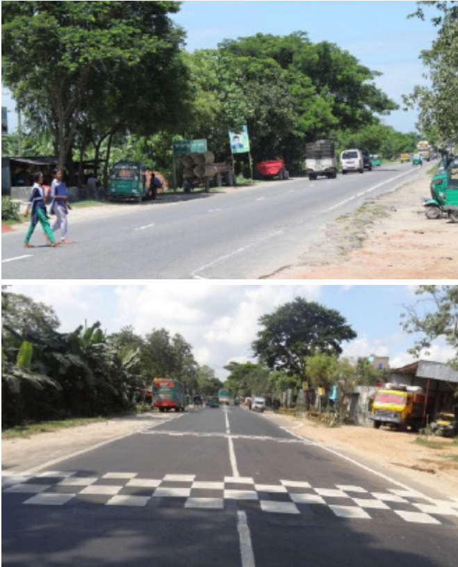
Figure 3.14: Installing speed table with checker marking. Left: before the intervention; Right: After the intervention.
