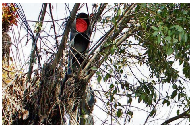
Figure 6.18: Signal hidden by the branches of a tree in Gurudwara, India; tree/branches must be removed or replace signal.
