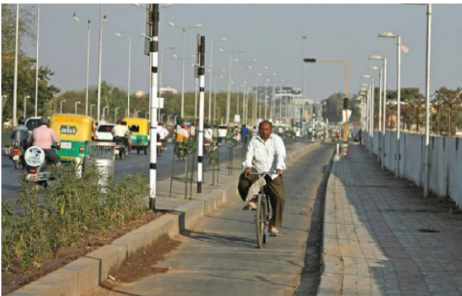
Figure 4.36: On-road segregated cycle path on a highway in Ethiopia.
