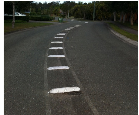
Figure 5.98: Median with pavement bars.
