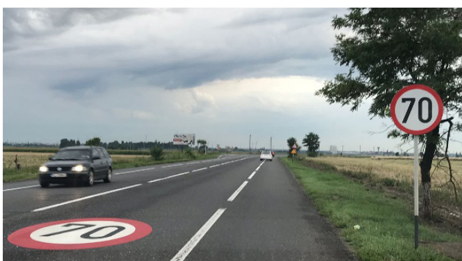
Figure 5.12: 2.5 m shoulder people wrongly using as a traffic lane—Romania.
