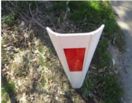
Figure 5.74: Lightweight guidepost that is forgiving.
