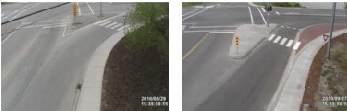
Figure 6.60: Angle of slip lane transformed from wide (left picture) to tight (right picture)
