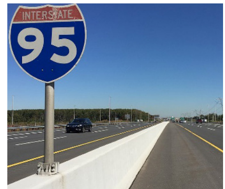
Figure 5.82: Rigid (F-profile) barrier.
