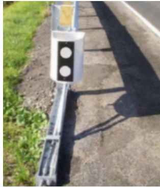
Figure 5.92: Fully re-directive terminal, flared or tangential.
