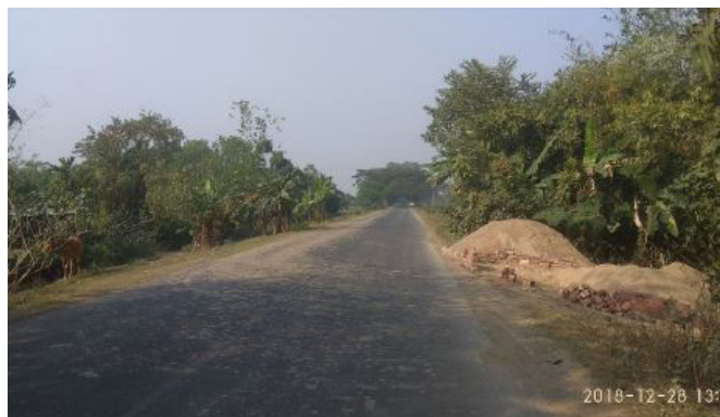
Figure 5.71: Stacked materials by the roadside. These are a particular hazard to two or three wheelers especially at night.
