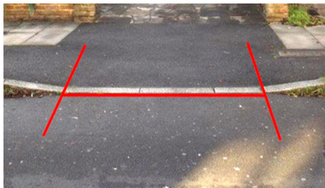
Figure 5.156: Dropped curb providing access to property.
