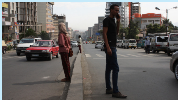
Figure 5.117: Narrow unsafe median
