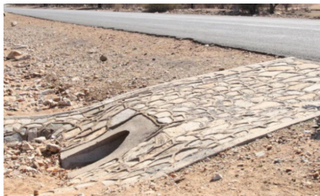
Figure 5.132: Typical extended culvert and revised headwall design.
