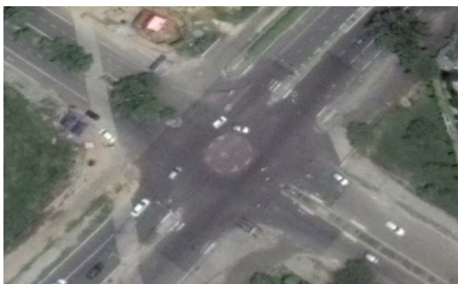
Figure 6.34: Roundabout with too small center island in India.
