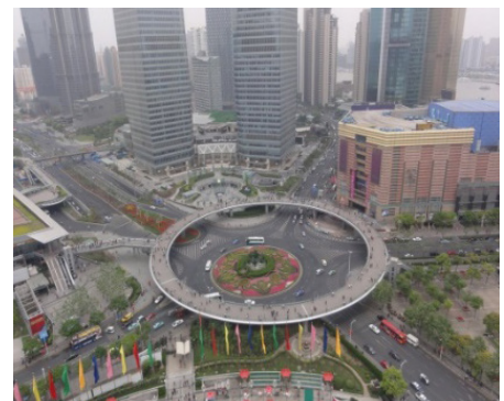
Figure 4.17: Well designed foot bridge—Shanghai.
