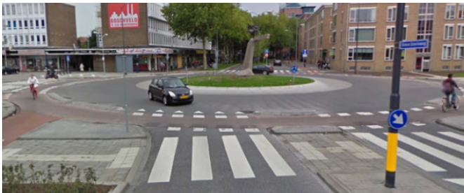
Figure 4.44: Roundabout for cyclists—Netherlands.
