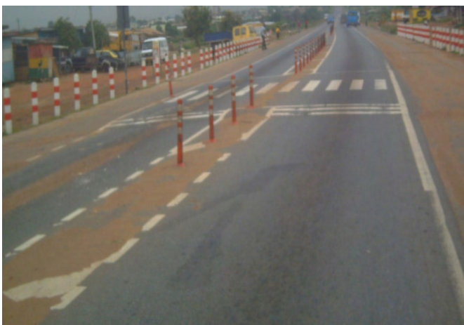
Figure 3.2: Carriageway narrowing, delineators, and speed humps.
