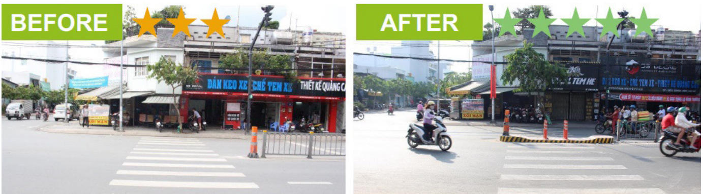
Figure 4.28: Installing pedestrian refuge—Vietnam.
