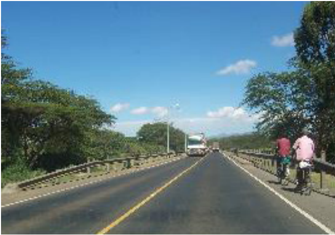
Figure 4.32: Cyclists using a narrow shoulder—Rwanda.
