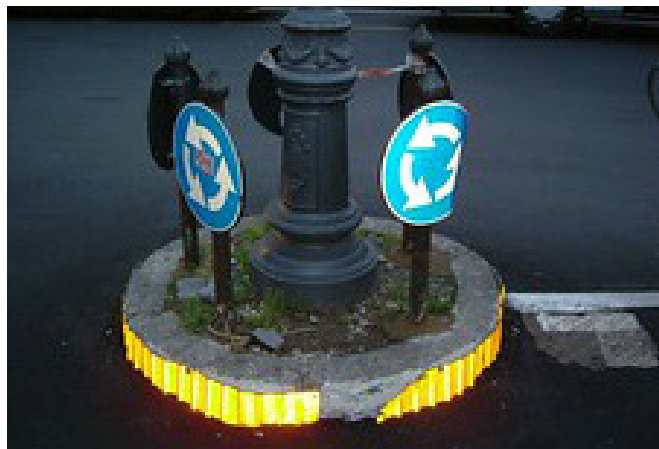
Figure 6.47: Example of mini-roundabout with reflection in Italy.
