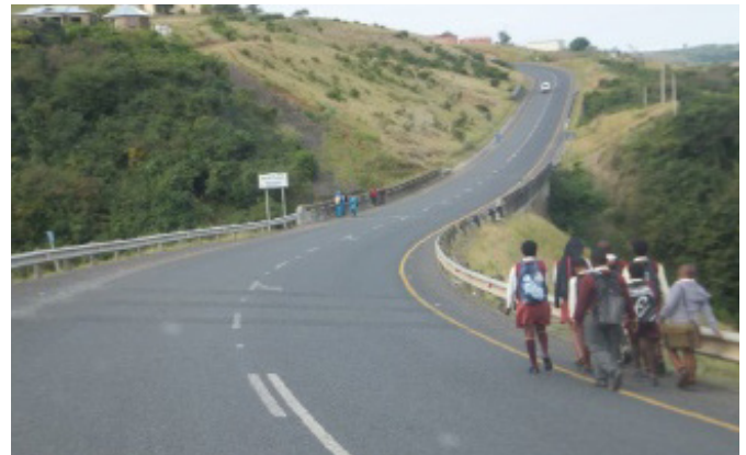
Figure 4.11: Unprotected footpath on rural national road.
