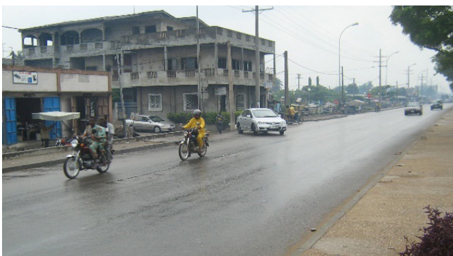
Figure 3.36: Local traffic not isolated from the expressway.
