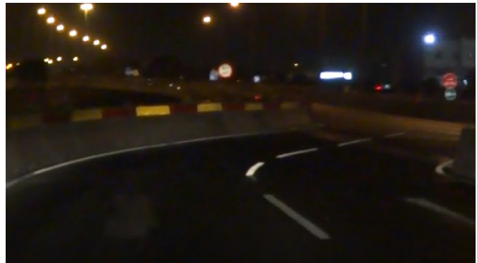
Figure 5.166: Line markings illuminated by retroreflecting material.
