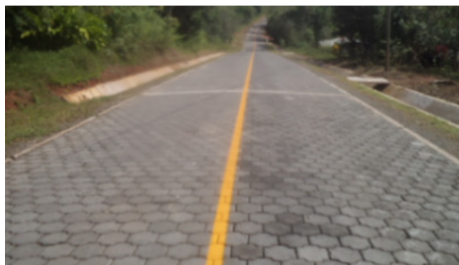
Figure 5.121: Concrete blocks (adoquines) surfacing in good condition and appropriate drainage facilities.
