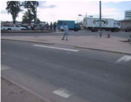
Figure 6.61: No marking slip lane in Tanzania.
