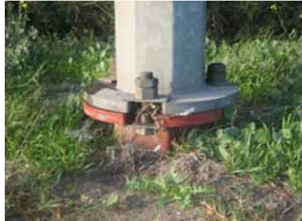
Figure 5.75: Slip-base lighting column suitable for high-speed roads with little pedestrian activity and parking.
