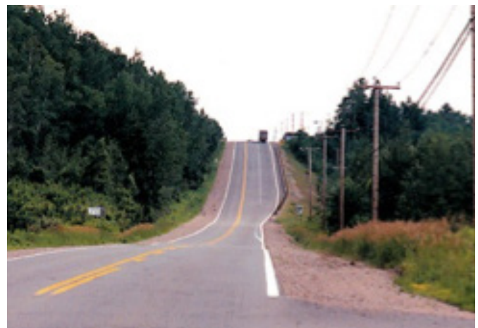
Figure 5.56: Example of markings on a climbing lane.
