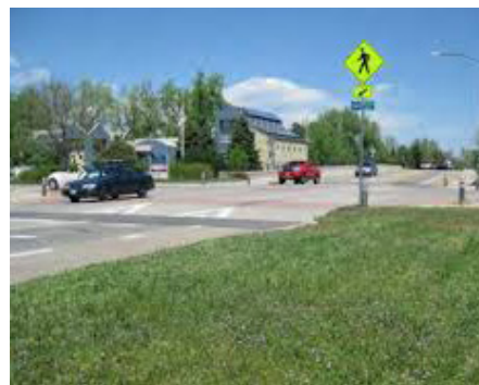
Figure 6.53: Raised intersection with crossing sign.
