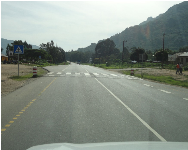
Figure 3.9: Marked speed hump for traffic calming
