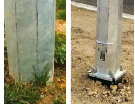
Figure 5.76: Impact-absorbing lighting columns suitable for low-speed
