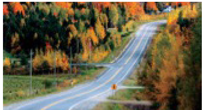
Figure 5.21: Hazardous combination: crest curve preceding sharp horizontal curve, with intersections and accesses.
