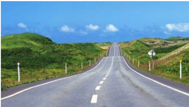
Figure 5.20: Poor alignment combination showing optical breaks caused by steep sag curves along horizontal tangent.
