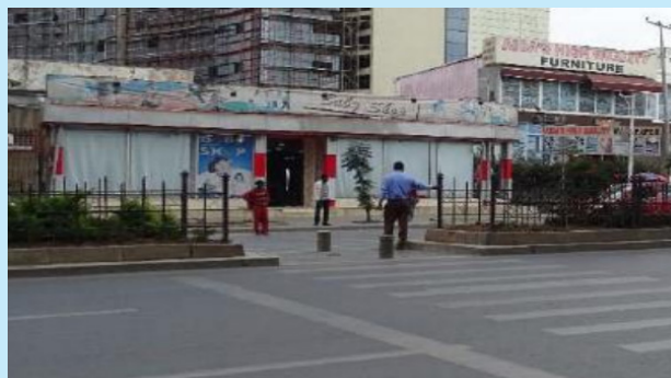
Figure 5.118: Wide median opening with concrete stumps
