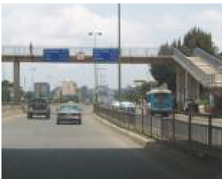
Figure 4.15: Grade separated footbridge—Ethiopia.
