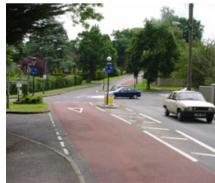
Figure 5.125: High friction surface (colored) applied on the approach to a mini roundabout.
