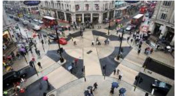
Figure 4.19: Scramble Intersection.
