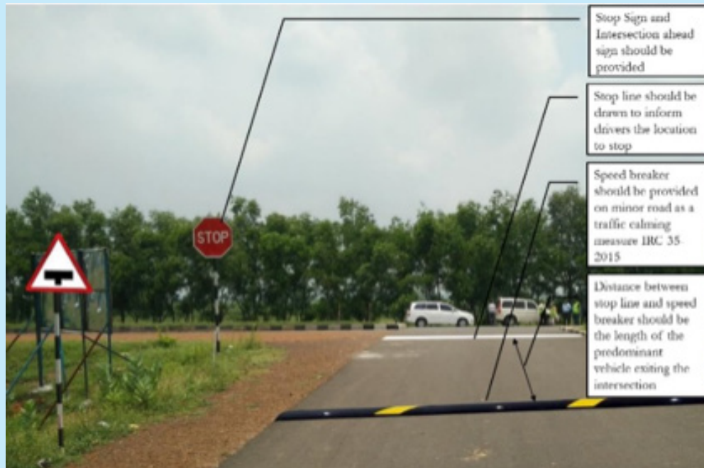
Figure 6.12: Minor road treatments—traffic calming and warning signs in India from minor road perspective.
