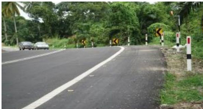
Figure 5.14: Wide, paved shoulder on curve.
