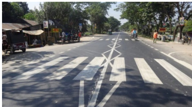
Figure 3.55: Well-maintained road with clear road markings—India.
