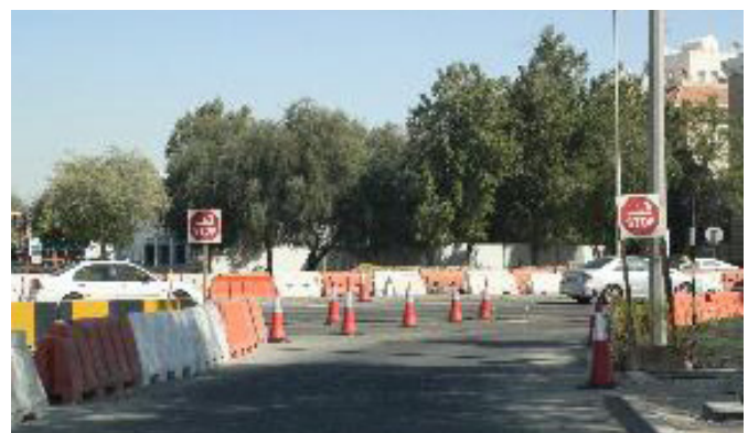
Figure 3.47: Well signed and guarded work zone—Abu Dhabi.
