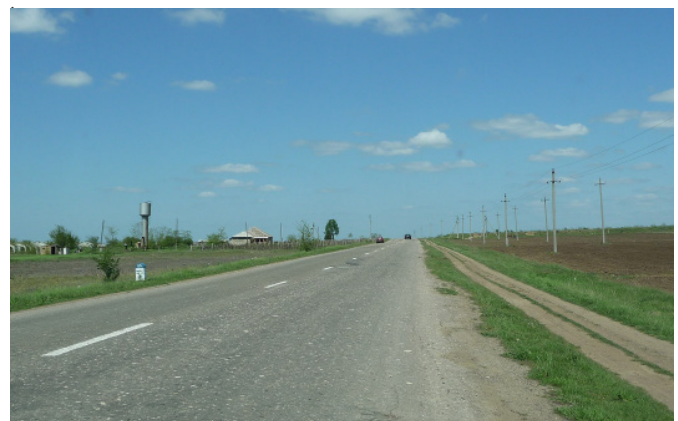
Figure 3.32: Moldova—service road for slow vehicles
