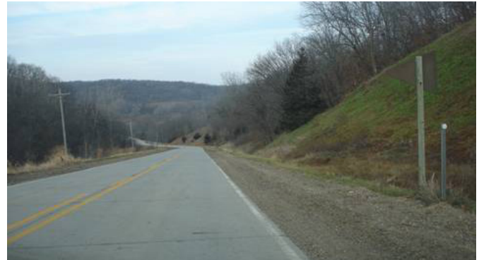
Figure 5.19: Hazardous combination of horizontal curve at the base of a steep upgrade.
