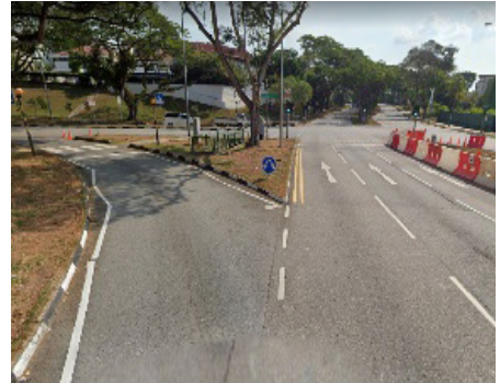
Figure 6.63: Slip lane with zigzag pavement marking in Singapore.
