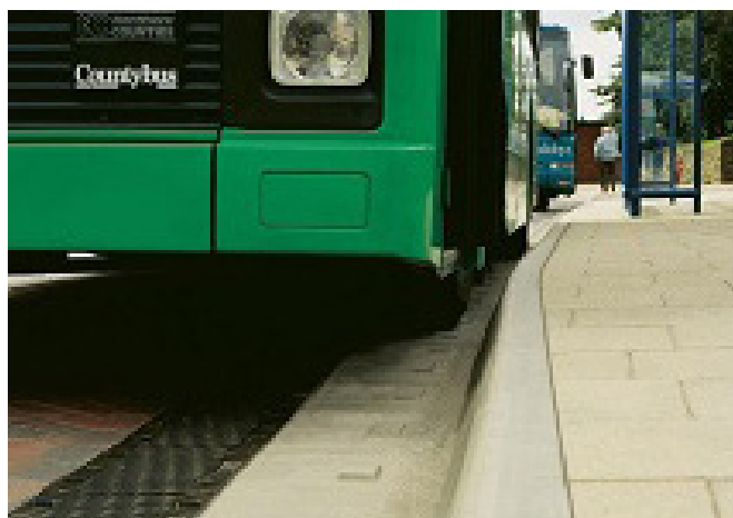
Figure 5.154: Bus-stop curb to ease passenger access.
