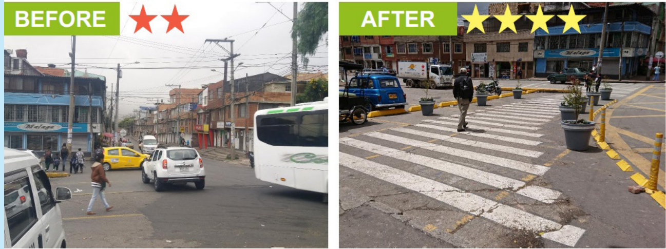
Figure 6.14: Installing movement prohibition measures and pedestrian protection measures—Colombia.
