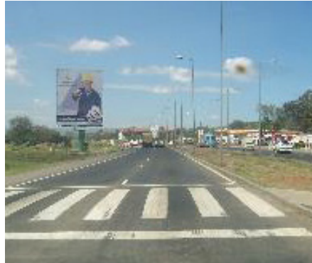
Figure 4.21: Raised crossing to slow approach speeds—Kenya.
