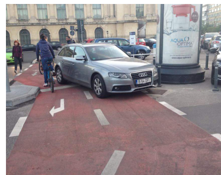
Figure 4.40: Unsuccessful cycle lane separated from vehicle traffic/parking—Bucharest, Romania.
