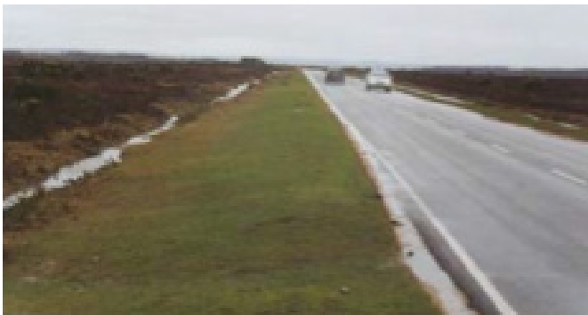
Figure 5.144: Safely widened shoulder and drainage.
