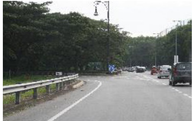
Figure 6.78: Deceleration lane approach tight exit radius—Brunei.
