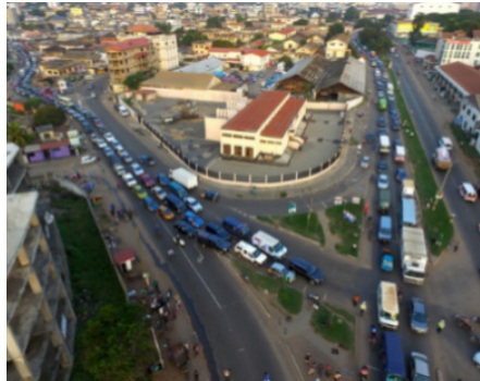
Figure 6.62: Poor delineated slip lane in Ghana.
