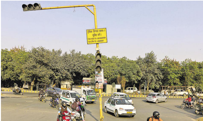
Figure 6.22: Intersection where signals are not functional in India
