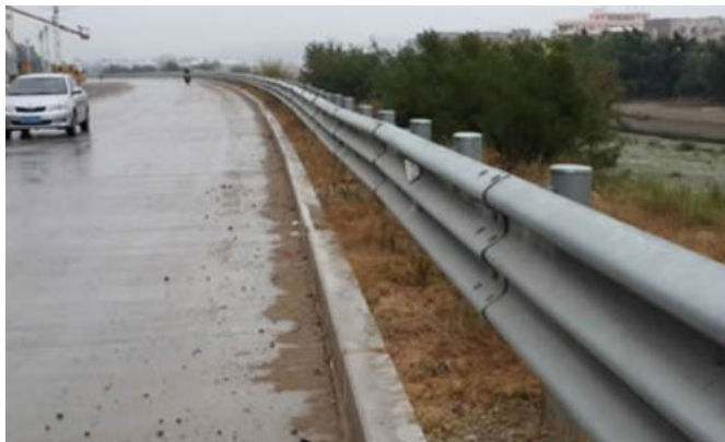
Figure 5.150: Example of dangerous curb-barrier combination with the steel barrier just behind the curb.
