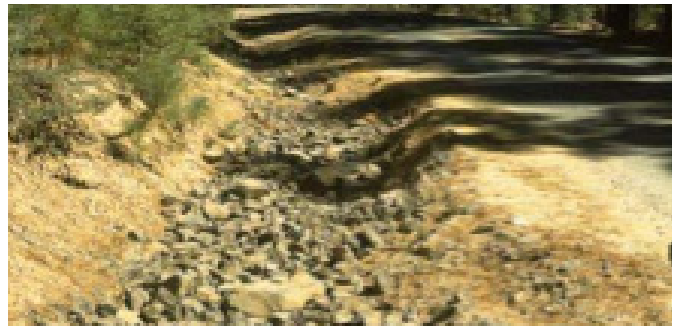
Figure 5.145: Armored roadside ditch with graded rock (riprap) for erosion control.
