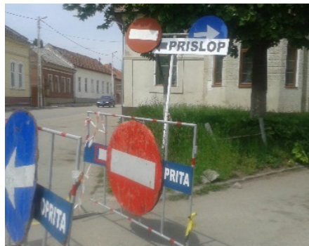
Figure 3.44: Uncontrolled signing—Romania
