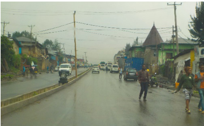
Figure 3.25: No footpath for pedestrians.
