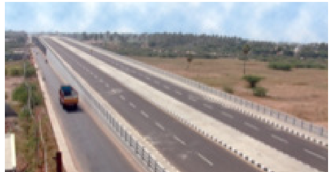
Figure 5.103: Raised median on dual carriageway.
