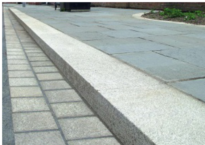
Figure 5.153: Vertical curb adjacent to footpath.
