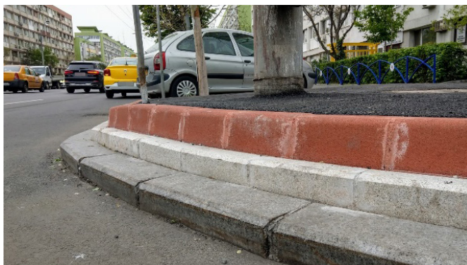
Figure 5.152: Triple curb in Bucharest, limiting access by pedestrians.
