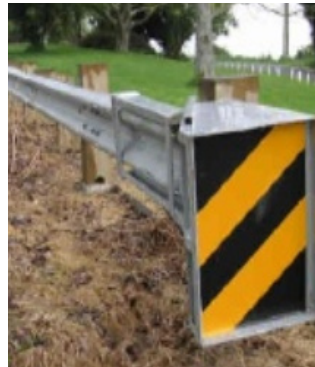
Figure 5.93: Flared energy absorbing terminal.
