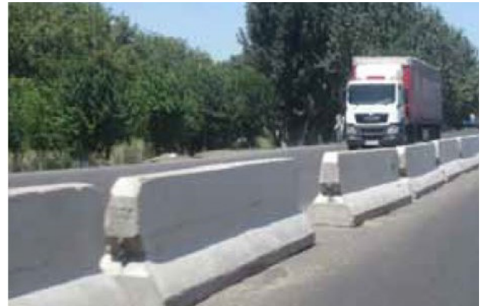
Figure 5.69: Individual concrete blocks.
