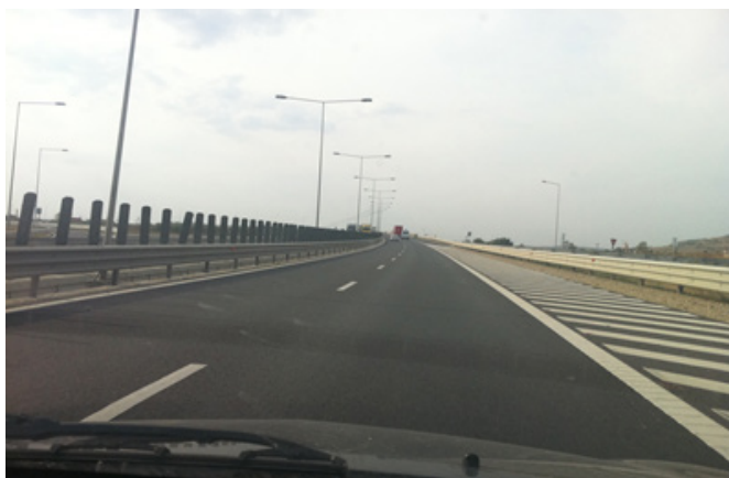
Figure 5.116: Anti-glare barrier on top of median.
