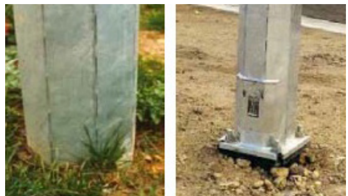
Figure 5.170: Impact-absorbing lighting columns suitable for low-speed environments with higher pedestrian activity and parking.
