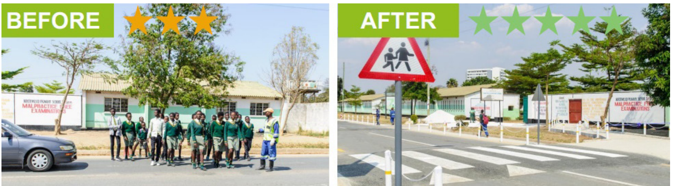
Figure 4.29: Installing raised crossing with signings and protected footpath—Zambia
