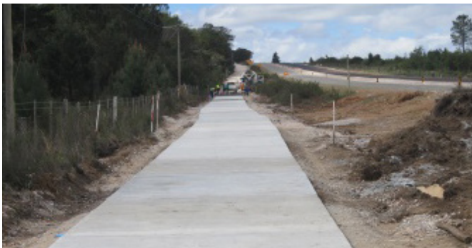
Figure 4.12: Segregated pedestrian/nonmotorized transport facility on rural road.
