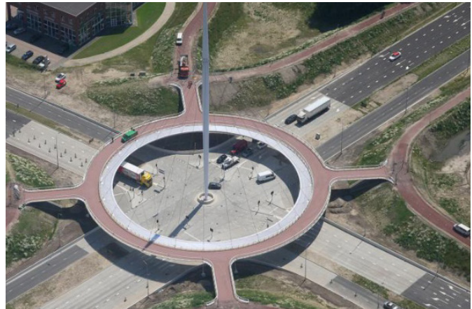
Figure 4.45: Floating roundabout for cyclists—Netherlands.
