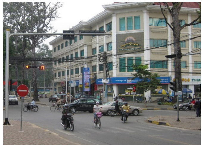
Figure 5.164: Faded pedestrian crossing markings in Cambodia.
