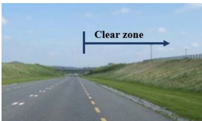
Figure 5.72: Example of a clear zone.
