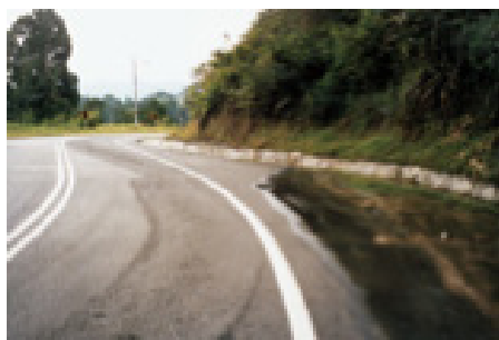
Figure 5.129: Wide paved shoulder and drainage facility on a downhill slope.
