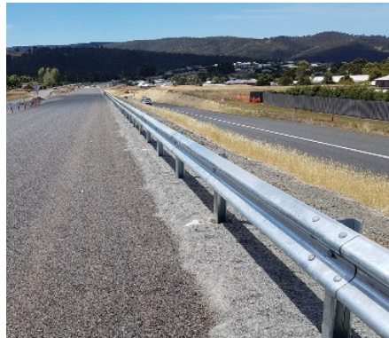
Figure 5.81: Semi-rigid barrier (W-beam).
