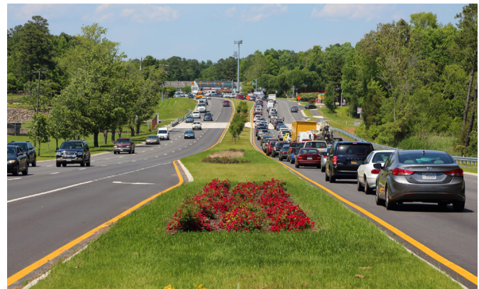
Figure 5.115: Raised median on carriageway.
