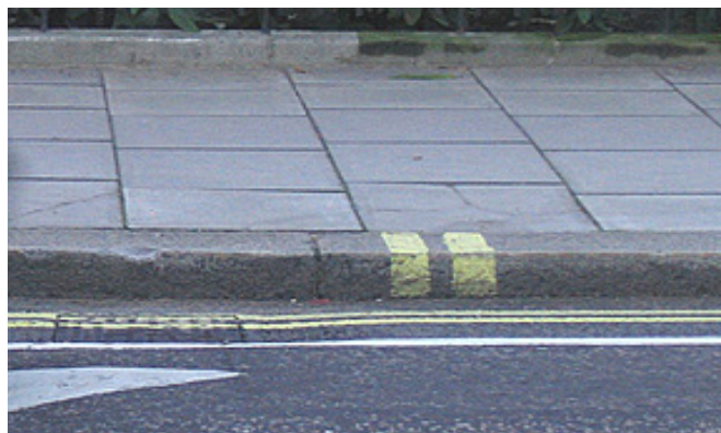
Figure 5.147: Concrete vertical curb.
