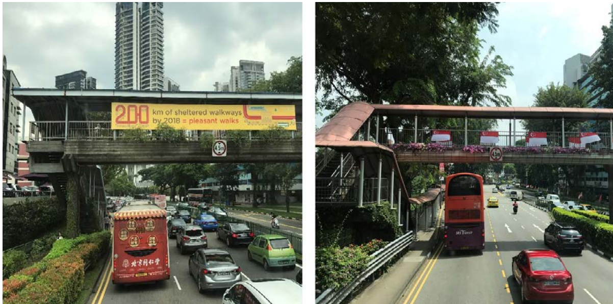
Photo 4.3. Examples of Frequently Used Footbridges in Singapore
