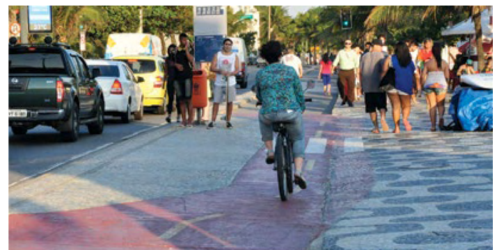
Figure 23. A bus station bypass in Rio de Janeiro, Brazil that raises the bicycle lane to the sidewalk level while bypassing the bus waiting area. Source: WRI
