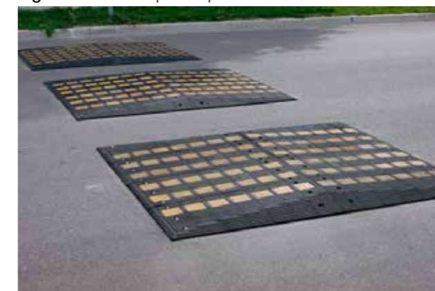
Figure 142 – Example of speed cushions
