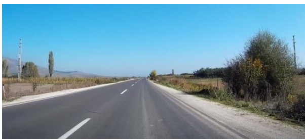
Too wide traffic lanes
