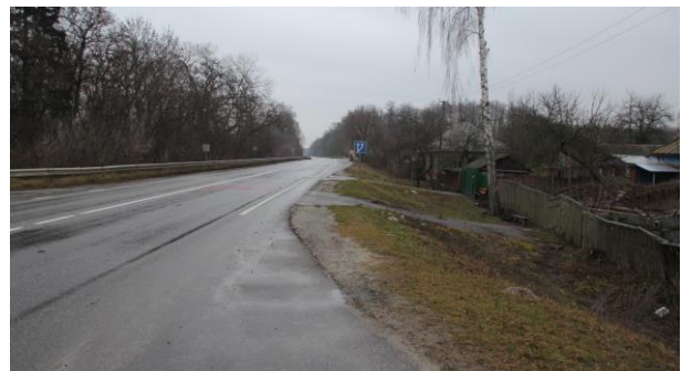
Missing of pedestrian footpath
