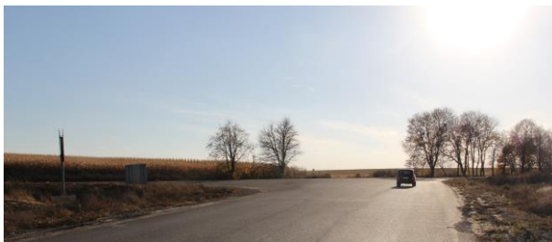
Insufficient orientation site distance at intersection
