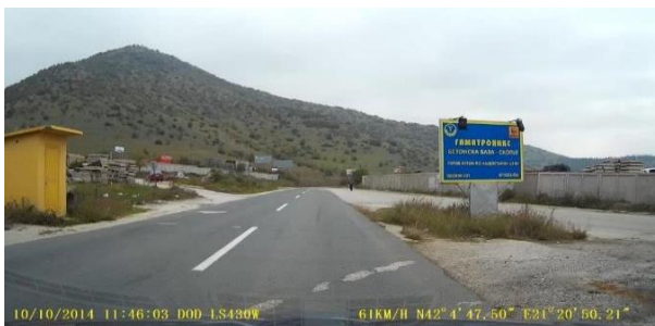
Missing access control
