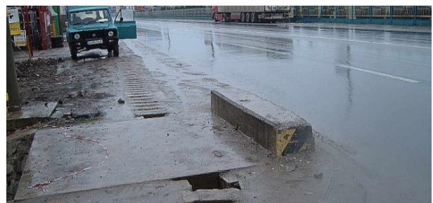
Drainage system as an obstacle
