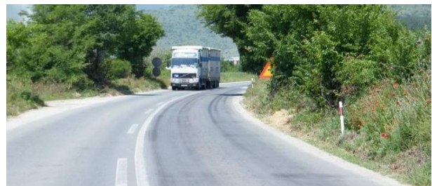
Insufficient stopping site distance in curve
