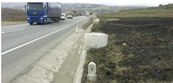
Drainage system as an obstacle
