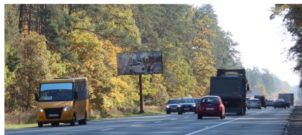
1+1 road with wide hard shoulders
