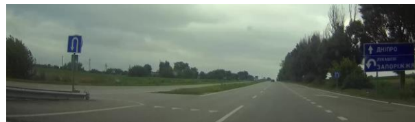
Unsafe solution of U-turn
