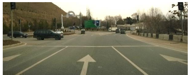
Missing channelisation in junction
