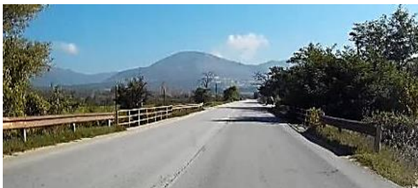
Dangerous guardrails (not a system)
