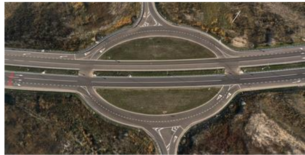
Unsafe solution of through roundabout "Hamburger"
