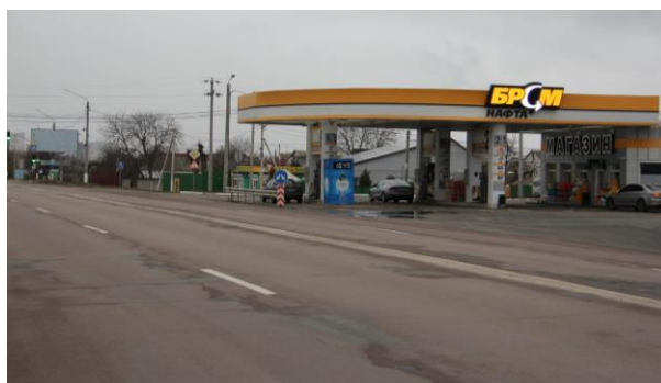
Services along road
