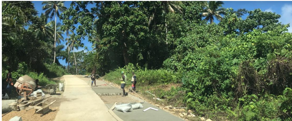
Photograph 6: Road under Rehabilitation (Mapillary 2018)
