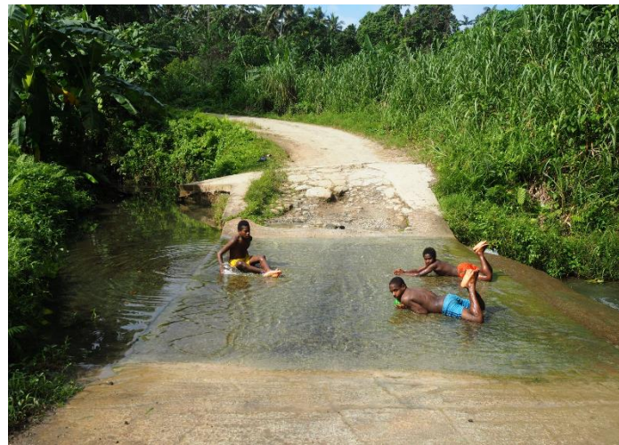
Photograph 8: Section of Santo Road (World Bank 2019)
