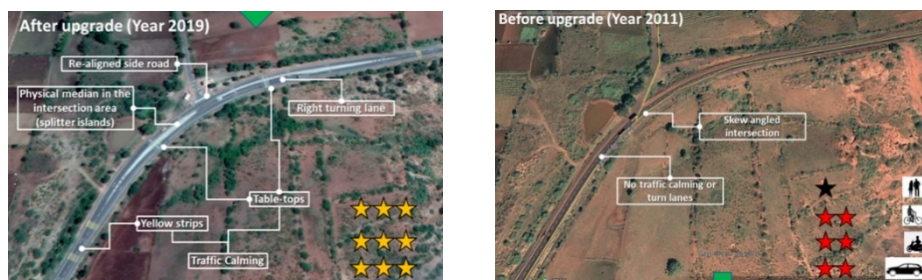
INTERSECTION IMPROVEMENT AT KM 46.9 RESULTING IN 3-STARS FOR ALL ROAD USE
