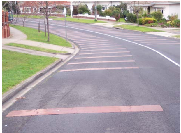
Maltravers Road, Ivanhoe
