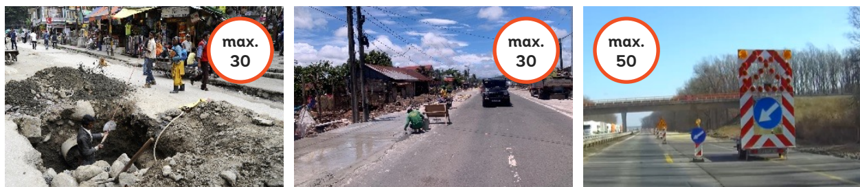
Figure 12. Typical examples of roadwork zones
