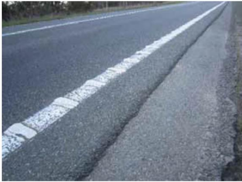
Figure A.11: Exemple de bandes d'avertissement sonore longitudinales (source: Secretariat CAREC 2018. CAREC Road Safety Engineering Manual 2: Safer Road Works)
