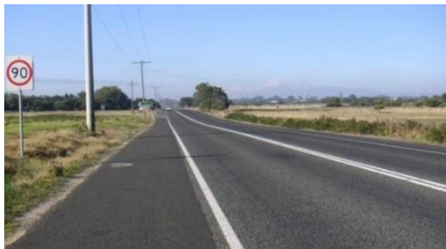
Figure 5.13: Large accotement scellé.
