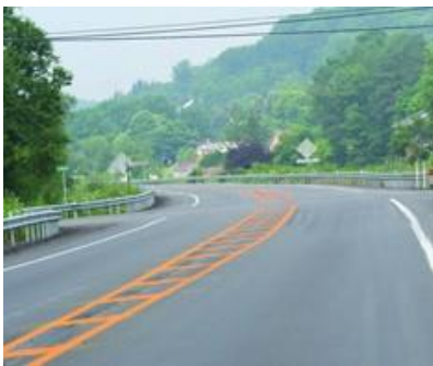
Figure 5.96: Terre-plein central affleurant.
