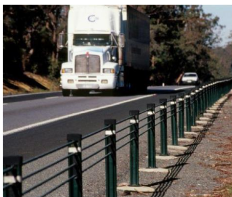
Figure 5.80: Glissière souple (câble).
