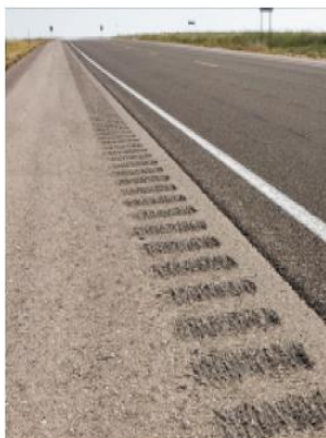
Figure 5.31: Bandes rugueuses aux accotements.
