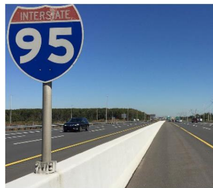
Figure 5.82: Glissière rigide (forme en F).
